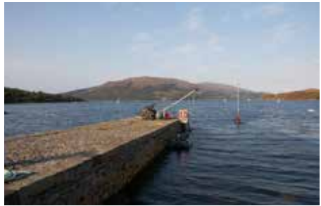
Pier at Isle D'Ornsay, Sleat, Isle of Skye, where some of the early emigrant ships left from Skye. Image: Lynda Collier.
